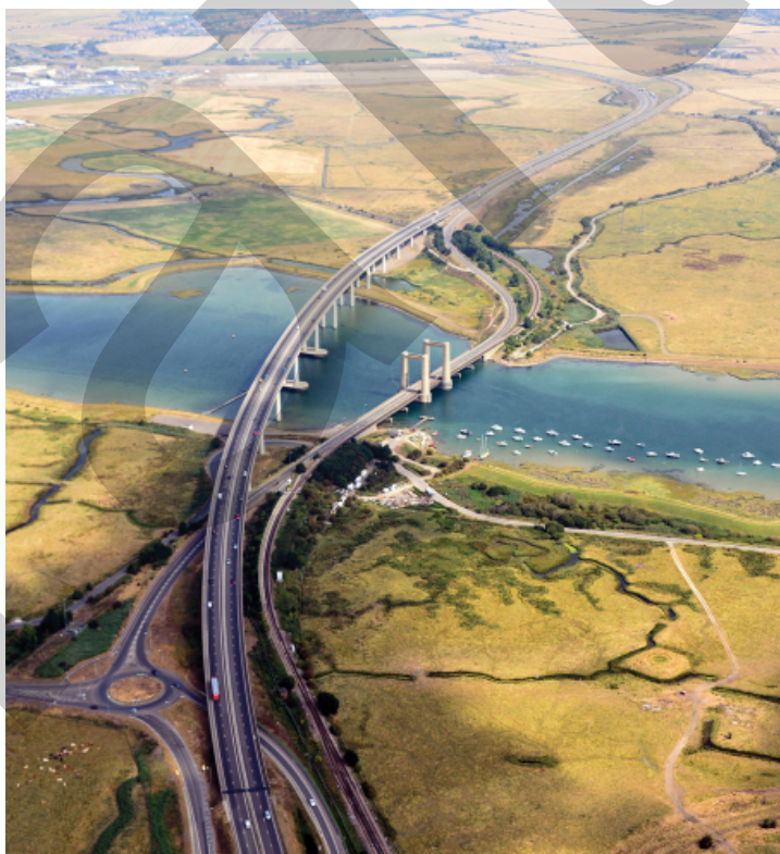
Picture 1.0.1 The Sheppey crossings
