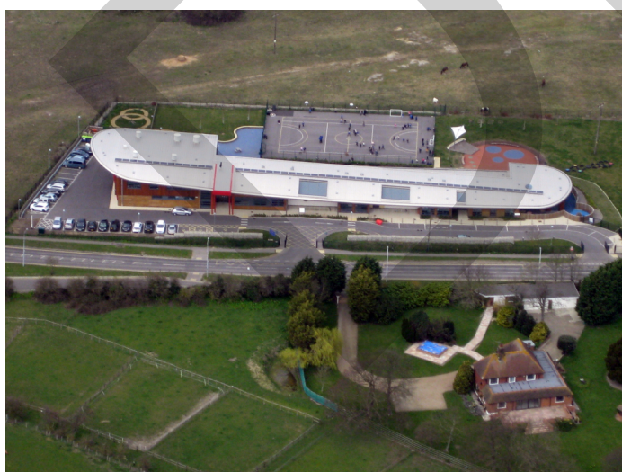
Picture 7.4.2 Primary school at Leysdown (SBC)
