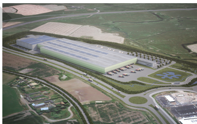
Picture 7.2.1 Aldi Depot, Queenborough (SBC)
